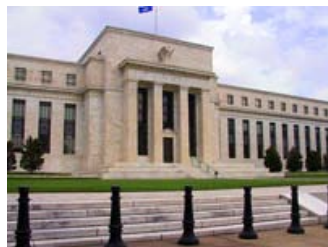
The Federal Reserve headquarters in Washington, DC.
