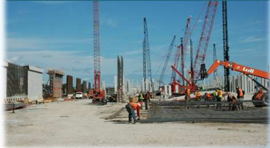
Runway Structures Bents (Walls) and Piles
