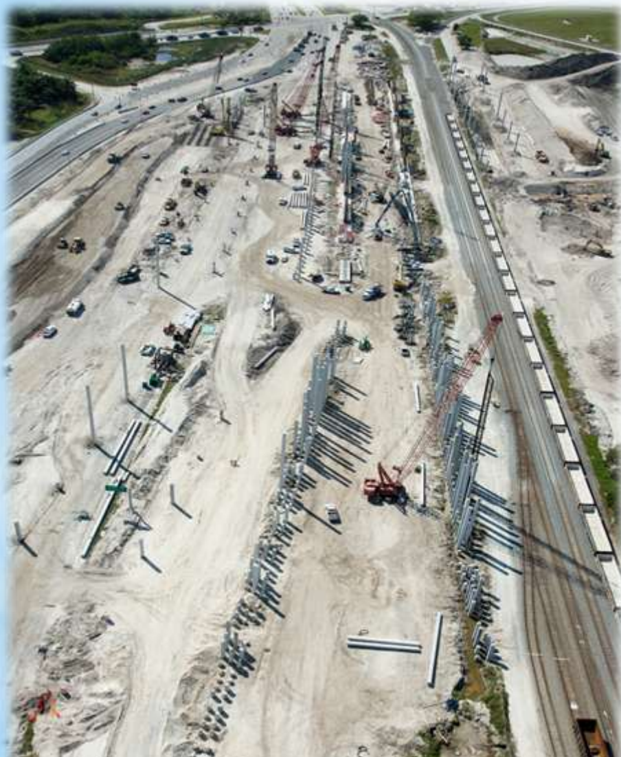
Runway Structure Piles, Utilities and Earthwork
